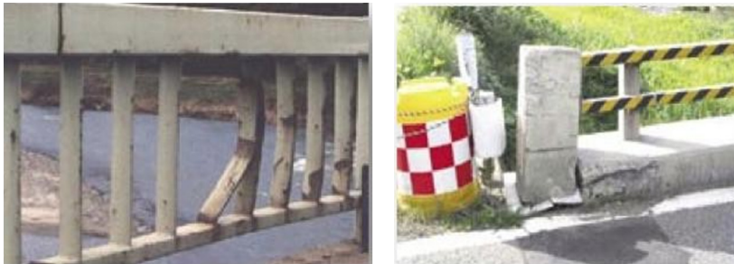
Figure 4-51: Image of Damage Railing
