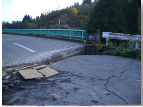
Figure 4-54: Depression of Road Surface at the back of the Abutment
