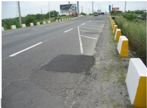
Figure 3- 11: A cracked patch which is rated as cracking and not patching followed by a successful patch which is rated as patch
