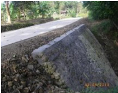
Figure 2-4-16: Grouted Riprap
