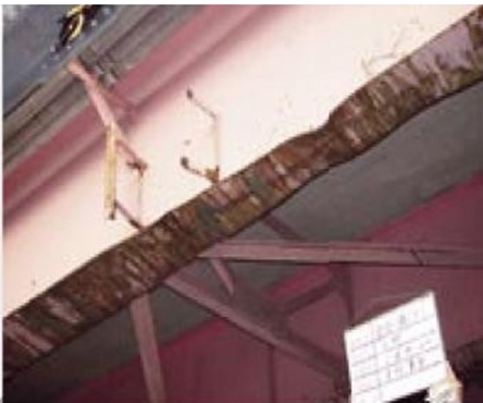
Figure 4-46: Damage and Deformation under the Girders
