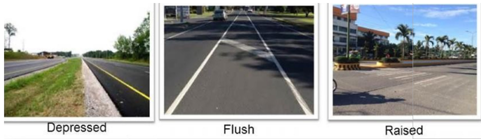
Figure 2-4-8: Surface and Pavement Description
