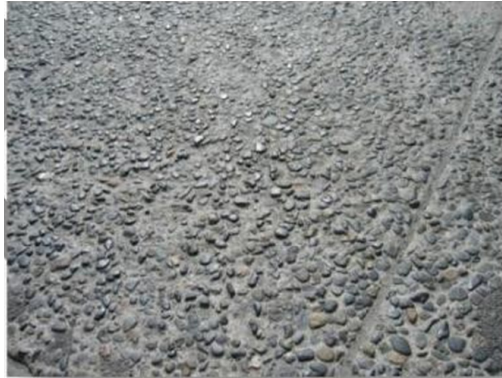
Figure 3-26: Example of Severe Scaling - rough texture
