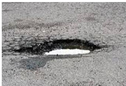
Figure 3-12: Example of Pothole
