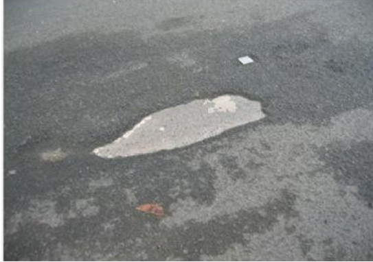
Figure 3-14: Surface failure due to delamination
