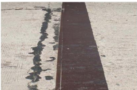
Figure 4-32: Steel Plate Slide Joint
