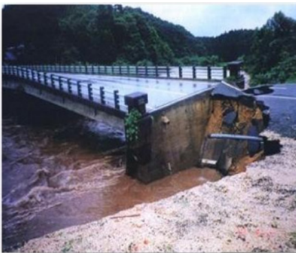
Figure 4-53: Washout at the back of the Abutment
