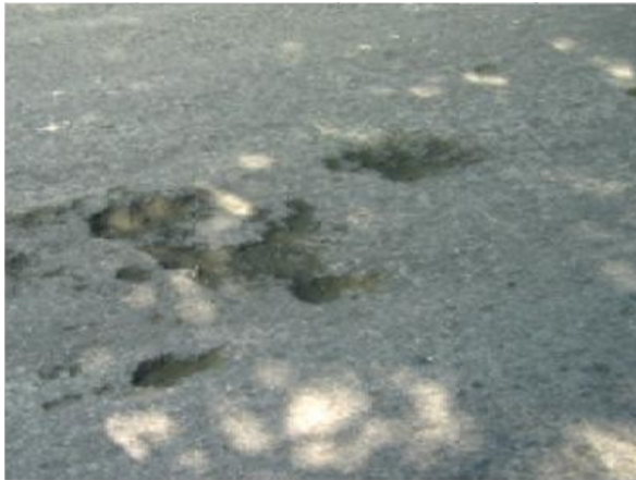
Figure 3-13: Example of Surface Failure due to wearing course deterioration
