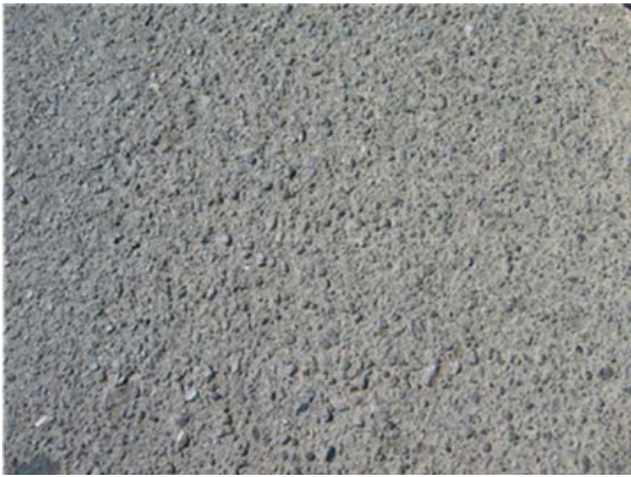
Example: Wearing coarse severe– coarse texture
