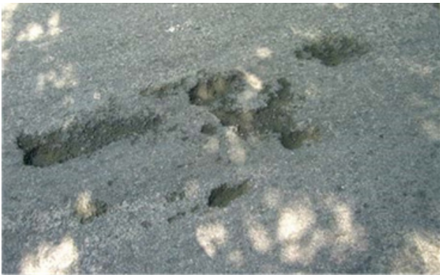
Example: Surface Failure, does not extend to unbound layer
