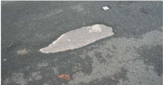
Example: Surface Failure due to delamination
