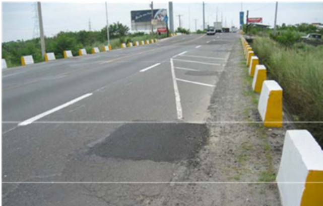
Example: A cracked patch which is rated as cracking and not patching followed by a successful patch which is rated as a patch.
