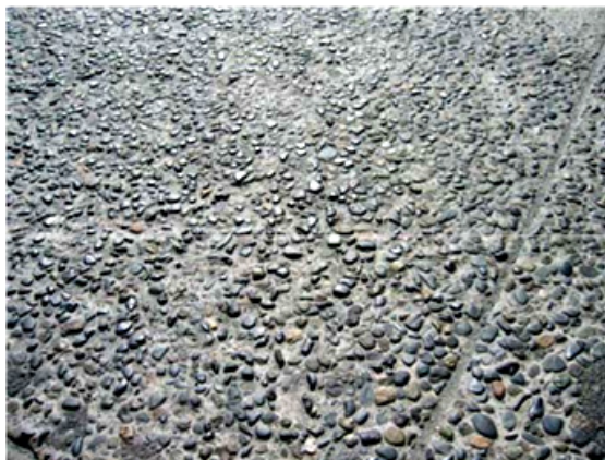
Example: Severe Scaling—rough texture
